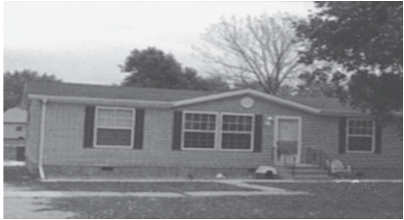
The Iowa Northland Regional Council of Governments received a grant from the State Housing Trust Fund and worked with the City of Hazelton to provide this new safe, affordable home to a terminally ill single mother and her two young-adult children, one of whom suffers from autism, after removing an unsafe dilapidated home.
