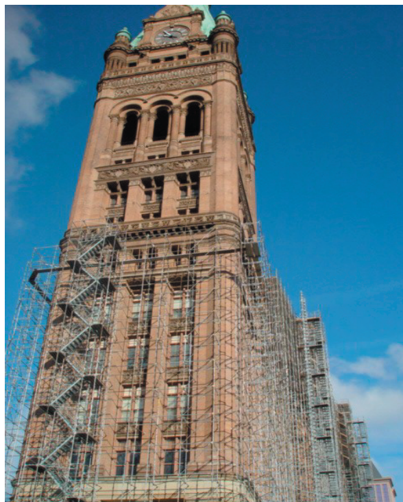
Renovation of the Milwaukee City Hall.
